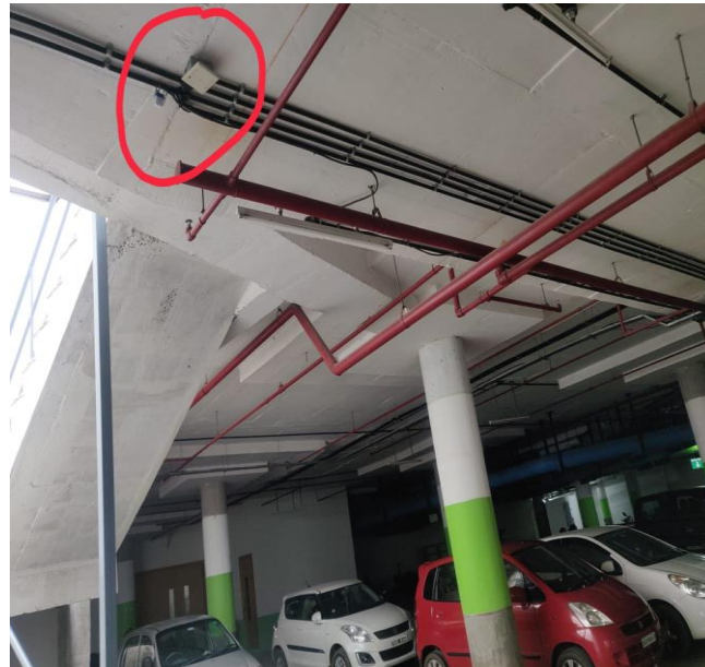
Additional 71 Movement Sensors & 2 daylight sensors installed, Saving 2300 Units
